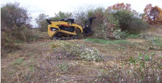
This is an invasive bush removal and Herbicide application job.
